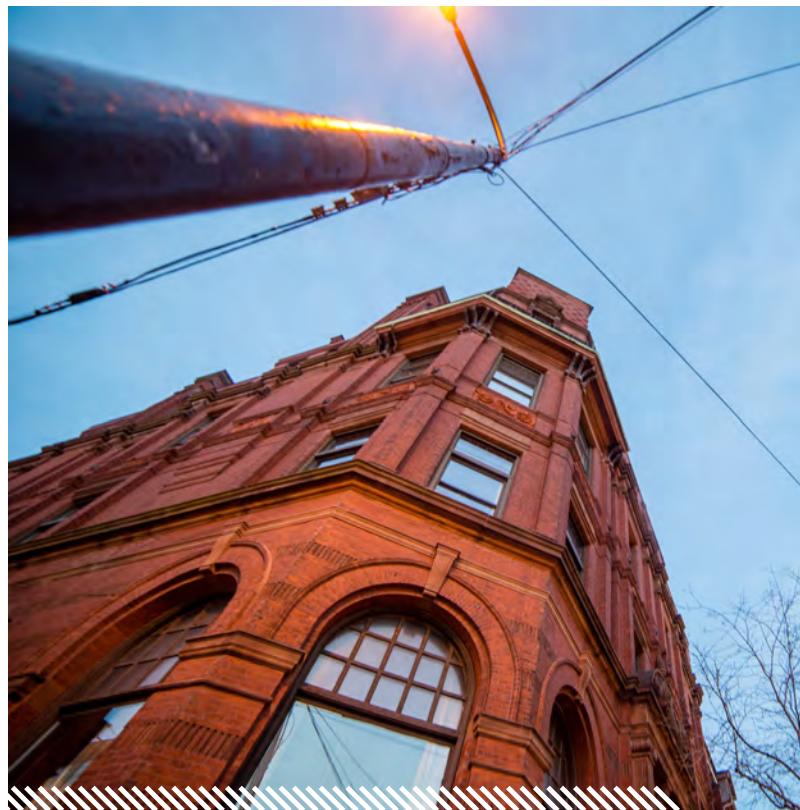
POWER LINES, CORNER OF MIDDLE AND EXCHANGE • Photo by Corey Templeton
